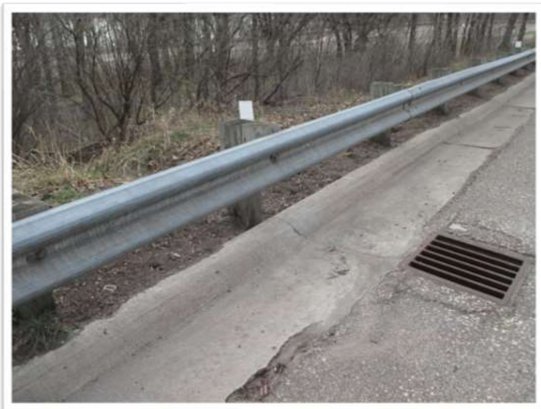
View toward southeast of existing right-of-way
