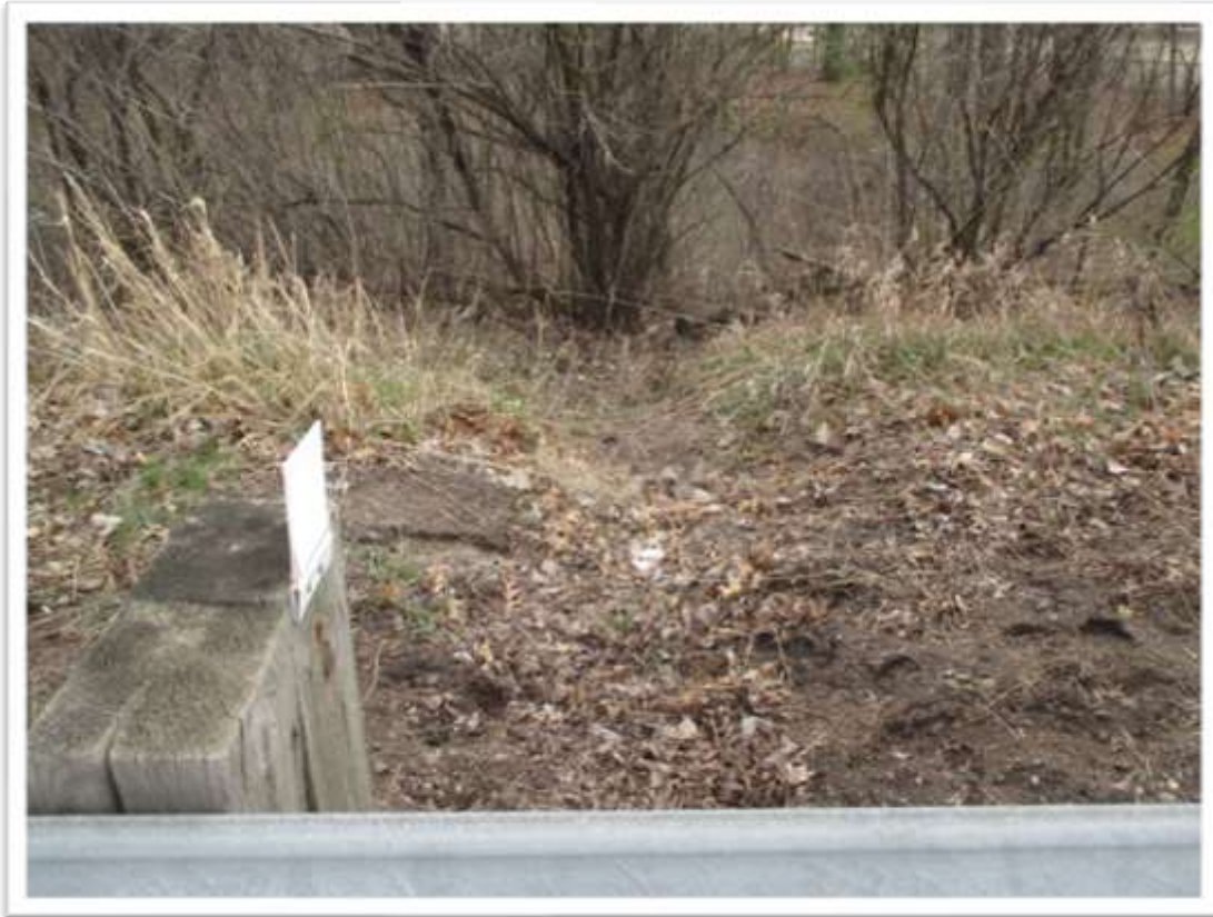
View toward acquisition facing east
