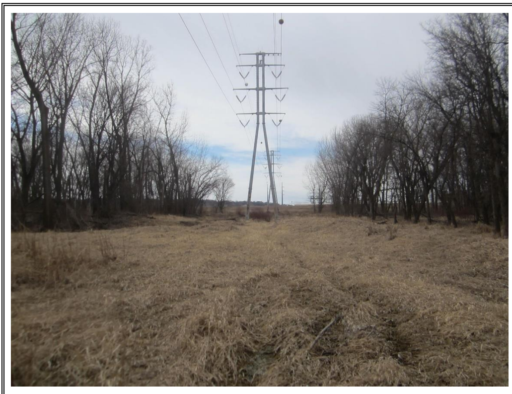
Looking Northeasterly at Powerline Easement Area of Subject Property from near West-Central Border of Site
