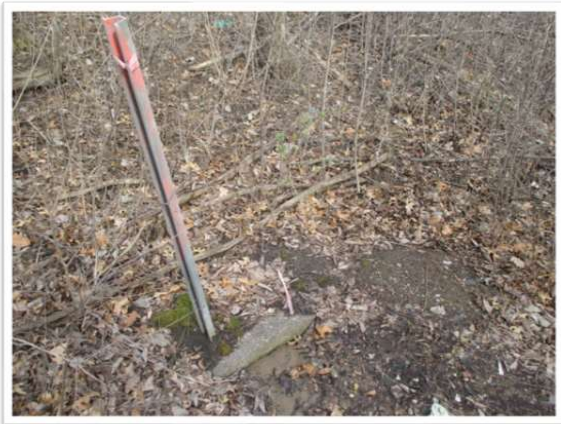
View of (clogged) existing drain apron
