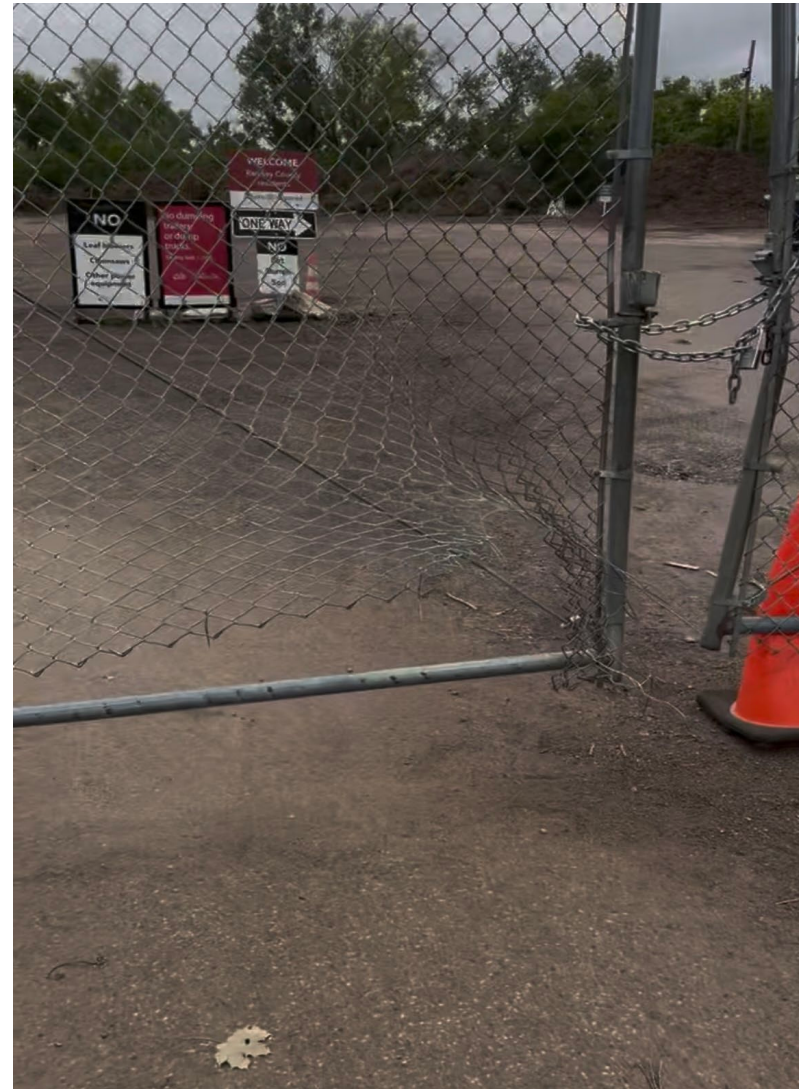
Photo of Midway Yard Waste Site
