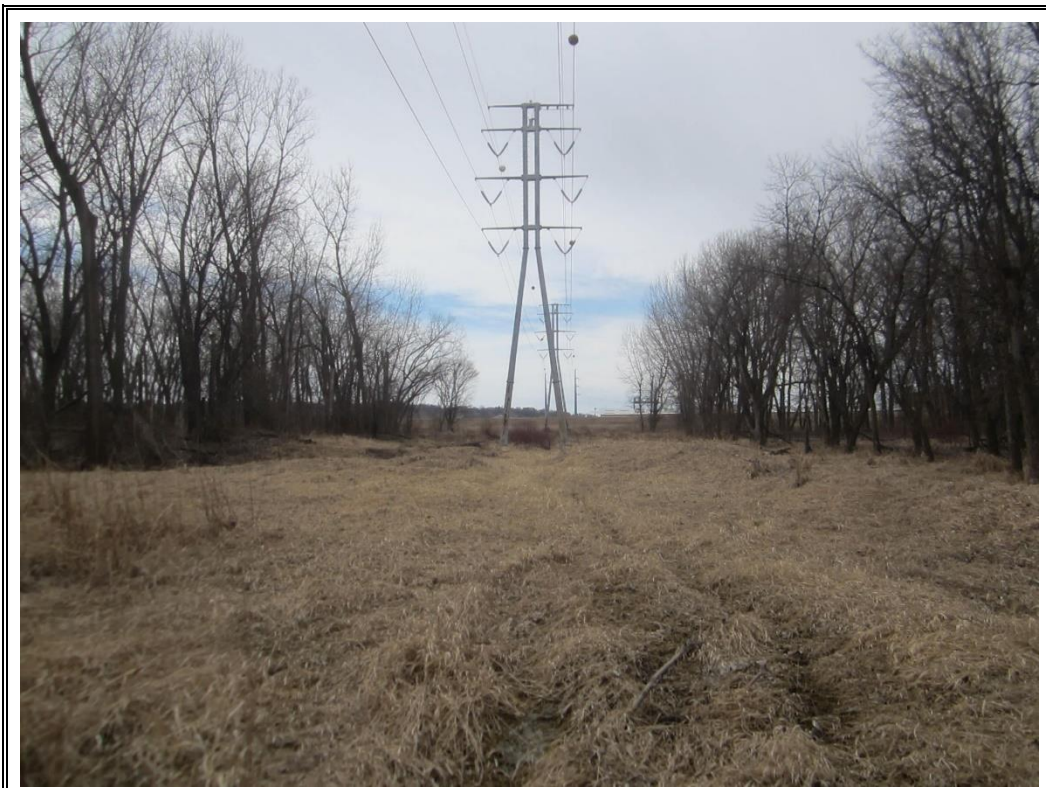
Looking Northeasterly at Powerline Easement Area of Subject Property from near West-Central Border of Site
